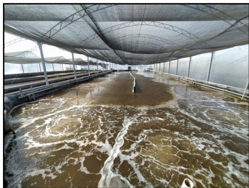
BFT System - Greenhouse
